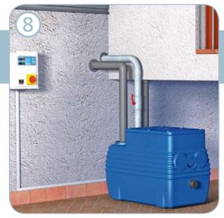
The BlueBOX lifting station is ready for use. The vast range of plumbing and electrical accessories covers all installation requirements.
