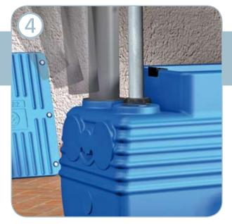
Once our BlueBOX has been placed in the installation position, the wastewater inlet and ventilation pipes are fitted.
